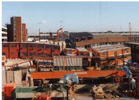
Heathrow tunnel collapse 1994 – Appropriate interpretation of instrumentation and monitoring data in a timely fashion was considered to be a contributing factor to the cause of the collapse
