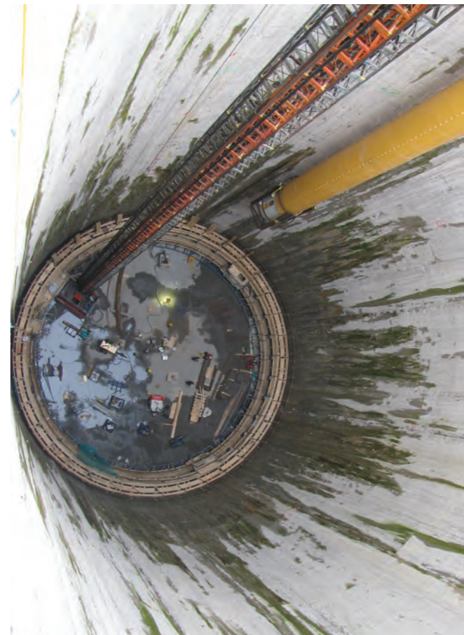
Deep circular diaphragm wall shaft – monitored with fibre optic instrumentation
