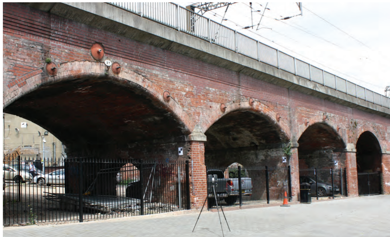
The monitored spans of the Victorian viaduct in Leeds
