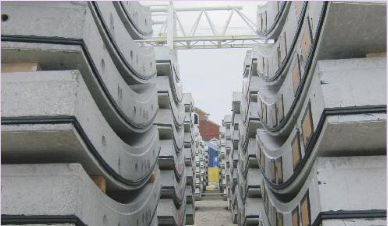
Tunnel lining segments awaiting installation in the National Grid Power Tunnel
