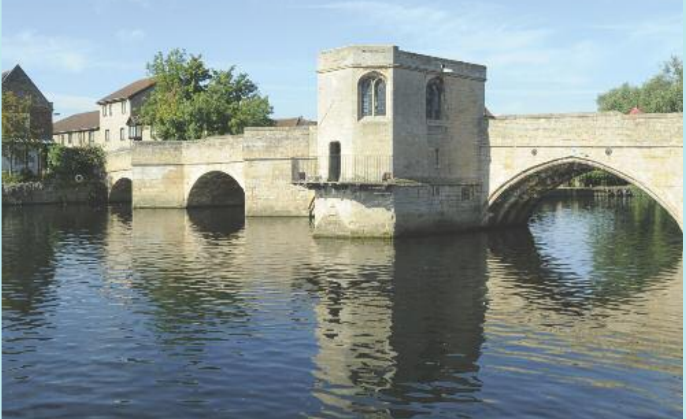
St Ives Bridge, Cambridgeshire, a fifteenth century bridge forming part of the CSIC and Cambridge County Council bridge maintenance portfolio. Picture courtesy of Cambridge News, Cambridge Newspapers Ltd
