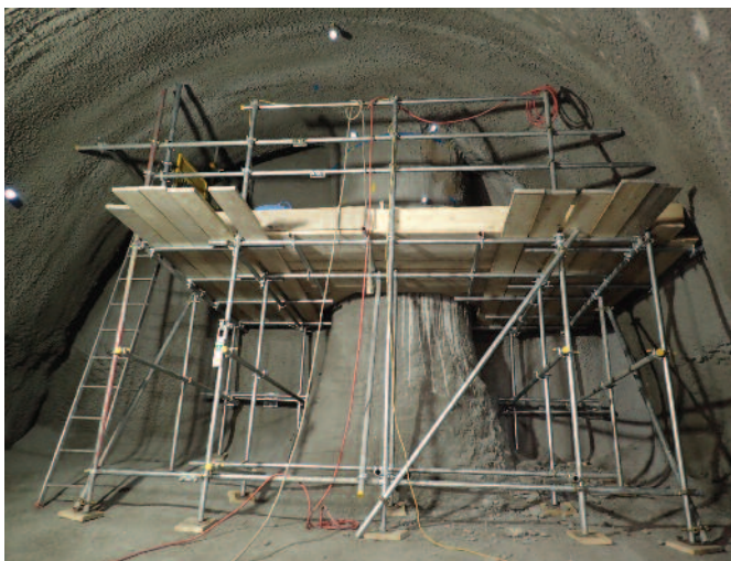
Figure 1: Exposed under-ream pile prior to cutting (TfL)
