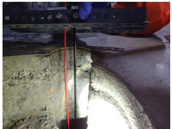
Figure 2: Fibre optic sensing cables being lower into cored pile
