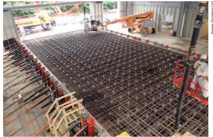
Figure 1: The strong floor instrumented with DFOS and FBG sensors being concreted
