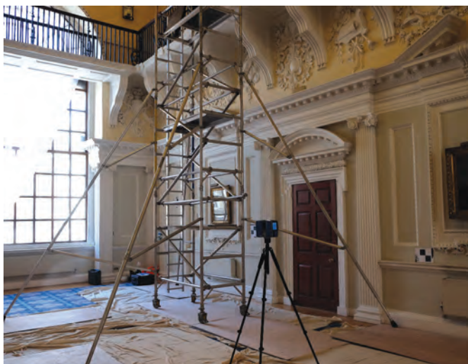
Laser scanning at Mansion House
