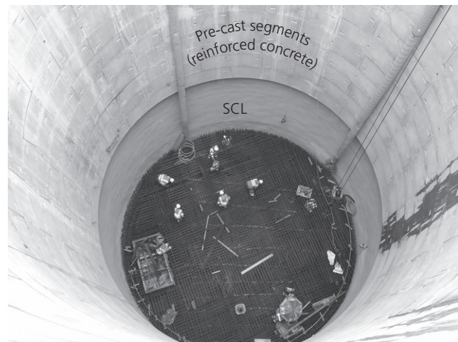
Figure 9. EBS shaft construction for National Grid's LPT project (NG, 2015)
