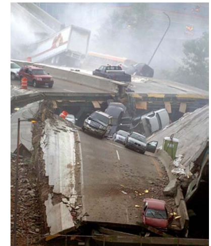
I-35 bridge collapse in MN (2007)
