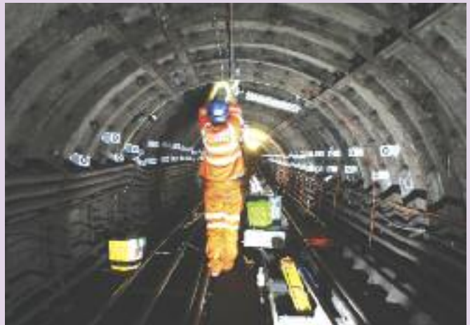
Filming of the installation of CSattAR photogrammetric technology in the Royal Mail cast iron tunnel, London
