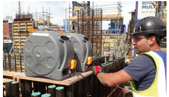
Operative installing fibre optic sensor cables
