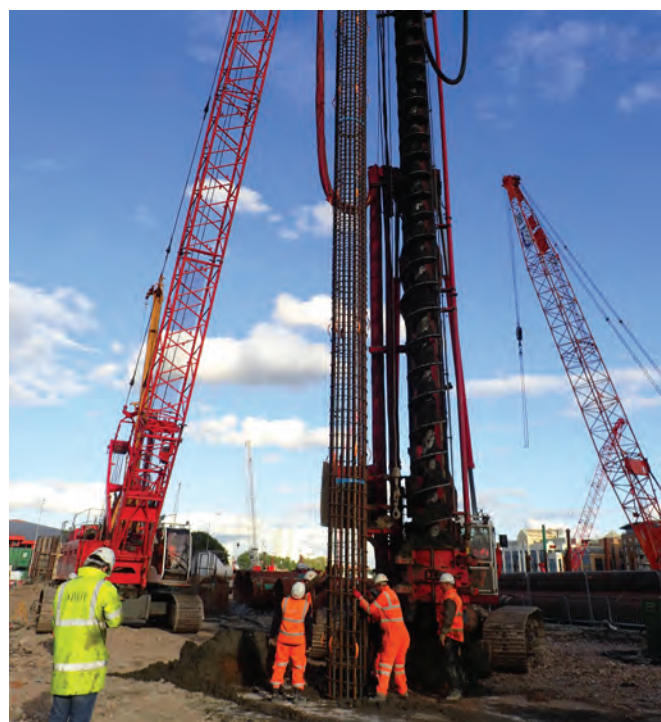
An instrumented CFA pile cage being inserted into the pile bore
