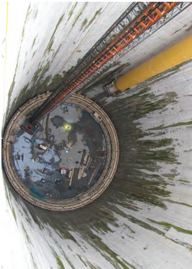
Deep circular diaphragm wall shaft – monitored with fibre optic instrumentation
