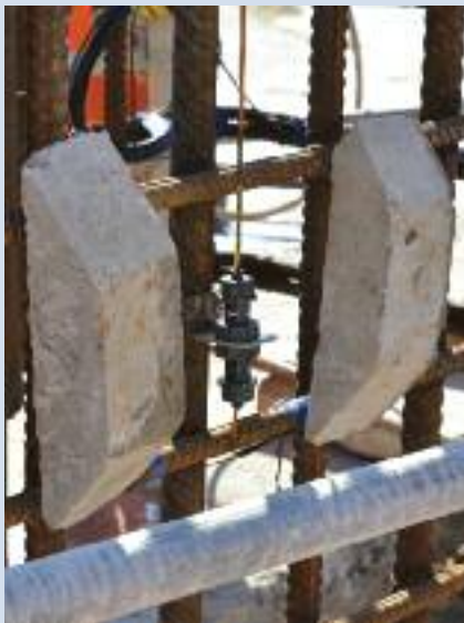
Attaching fibre optic cable on a diaphragm wall reinforcement cage
