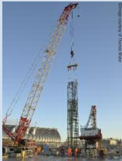
Installation of reinforcement cage with fibre optic cables
