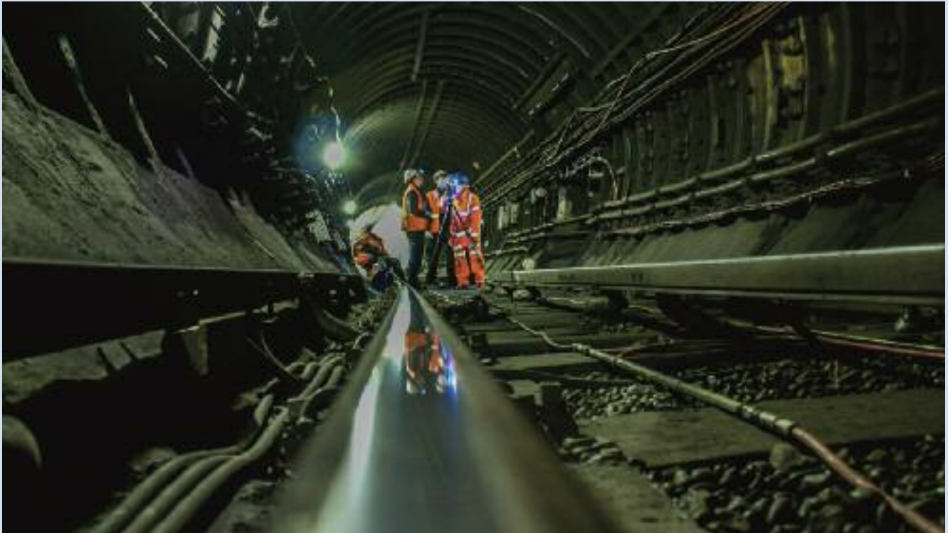
CSIC researchers with engineers from Tubelines surveying the tunnel geometry, feeding into London Underground's overall maintenance strategies
