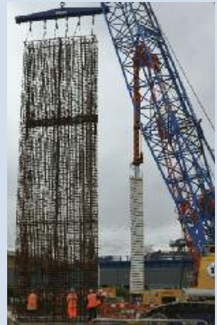
Above: installation of reinforcement cage for diaphragm wall with fibre optic sensors attached. Below: diagram showing detail
