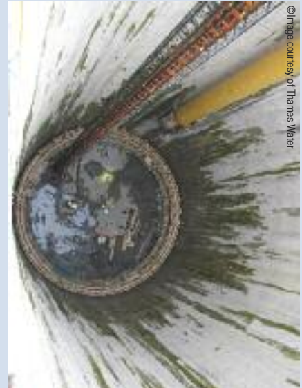
Deep circular diaphragm wall shaft – monitored with fibre optic instrumentation
