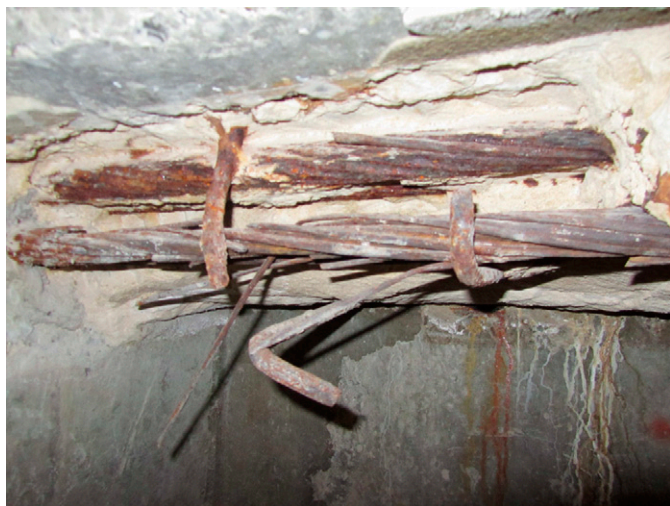
Fig. 2. Corrosion of prestressing tendons (image by authors, taken May 14, 2012)
