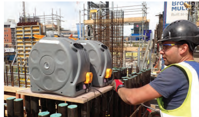
Operative installing fibre optic sensor cables
