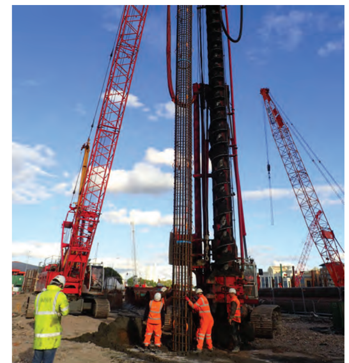
An instrumented CFA pile cage being inserted into the pile bore
