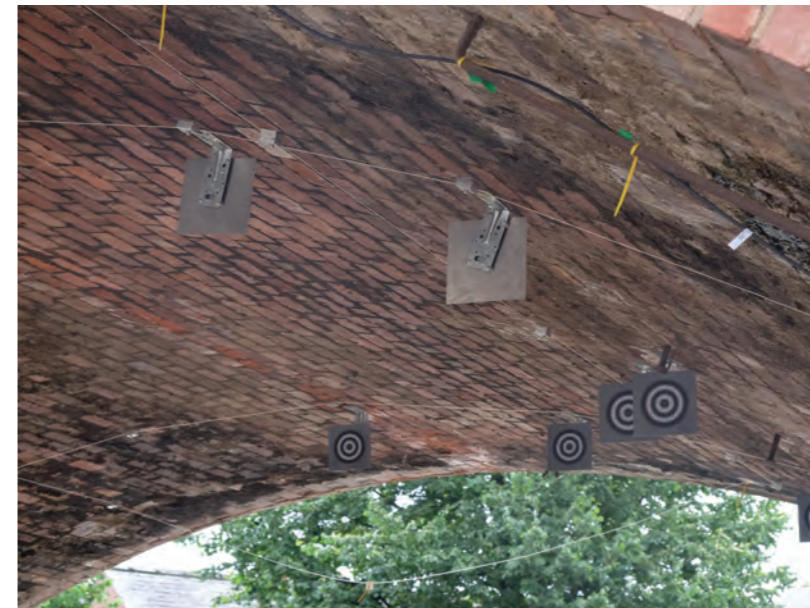
An arch instrumented with FBG cables and photogrammetry targets in the viaduct
