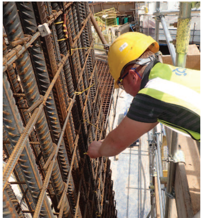
Figure 2. The fibre optic cables tied to the reinforcement prior to concreting
