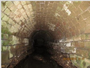
2164 - Marsh Lane Culvert
