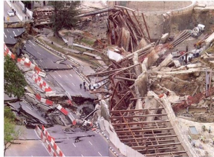
Metro station collapse Singapore 2004
